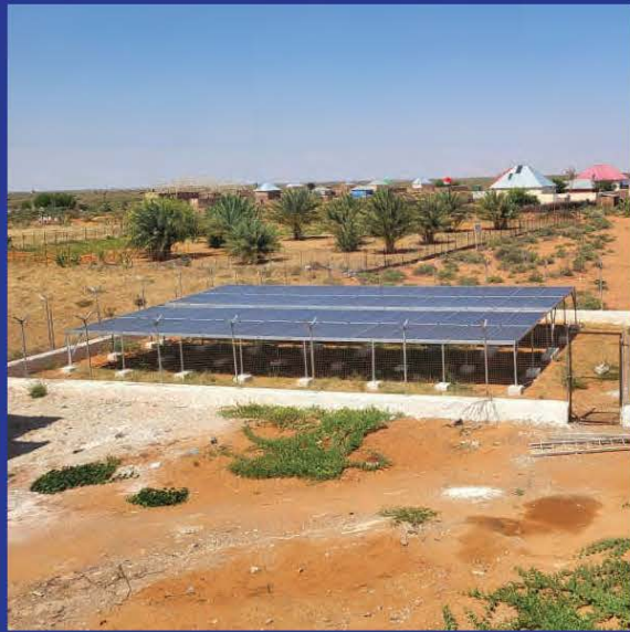
PUMP / SOLAR INSTALLATION FOR BOREHOLES
