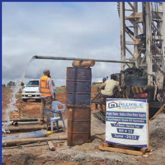
REHABILITATION BOREHOLES AND MAINTENACE
